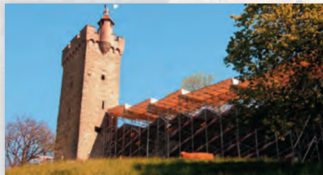
Restoration work 2004-2015 – last phase
